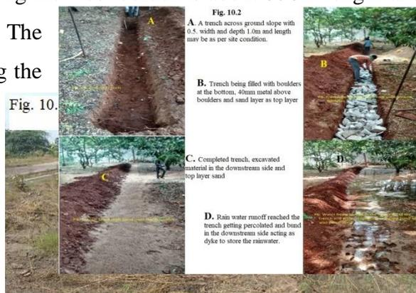
filled with sand to the top level. Instead of filling permeable material to the top level, top 25cm is to be left vacant to accommodate more water in the trench. Once in a year trench is to be maintained by removing the deposited silt and make it permeable.
